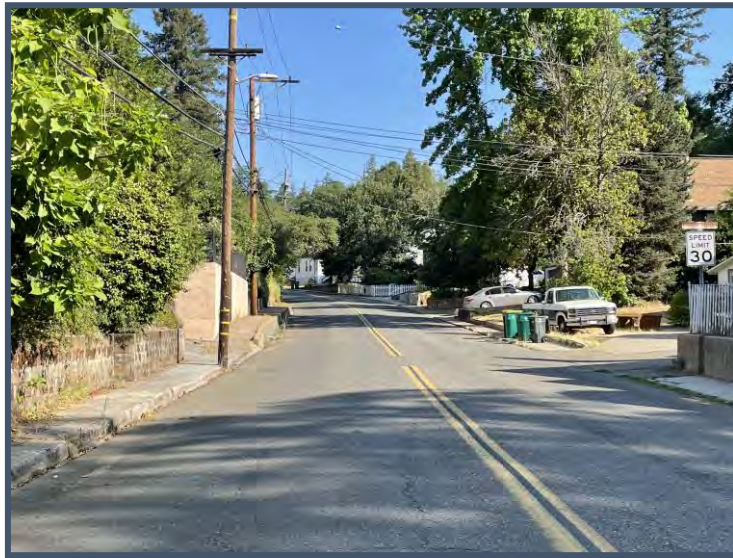
Image 1 – Canal Street looking northwest, view of elevated sidewalk and no gutter pans and utility poles encroach upon the already narrow sidewalk
