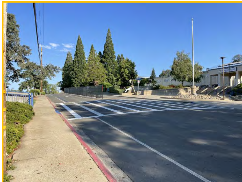
Image 2 – Canal Street along the High School, view of crosswalk with no curb ramps
